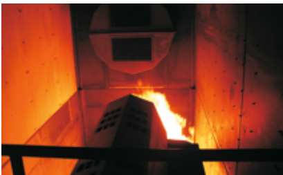
Motor and Boiler Fire
