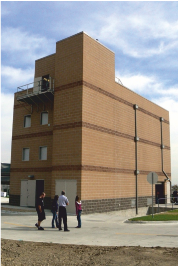
4-Story Training Tower
