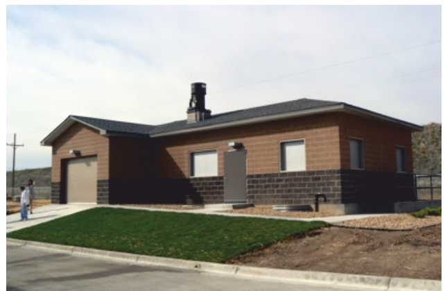
1-Story Residential Building
