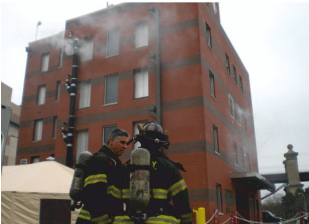
Structural FireTrainer® T-2000 Building
