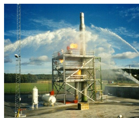
custom industrial fire
